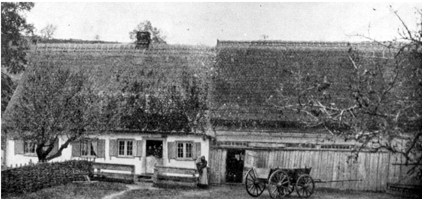
Figure 2. Mennonite housebarn on the Kamp of the Island of Chortitz, South Russia. Courtesy of the Mennonite Heritage Centre Archives, Winnipeg MB.
